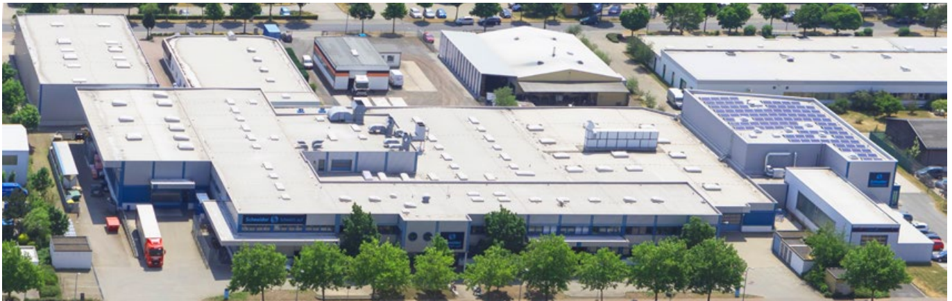
Production facility in Wernigerode
